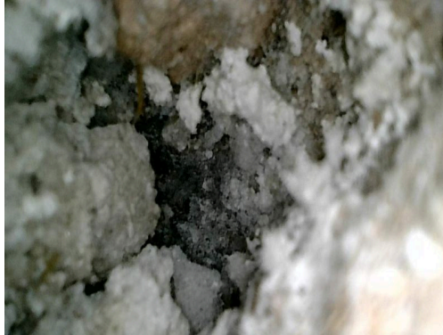
Photo indicators of filled cavity insulation:
