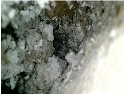
Photo indicators of filled cavity insulation:
