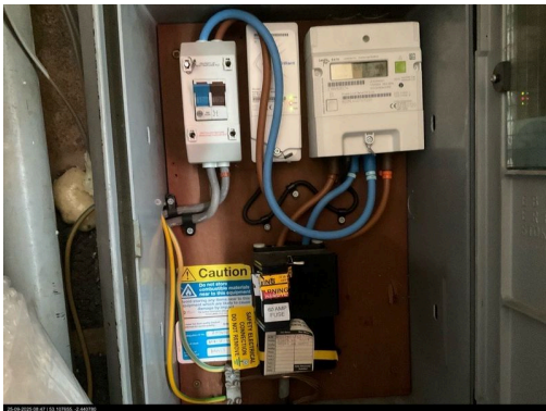
Photo of electricity meter:
