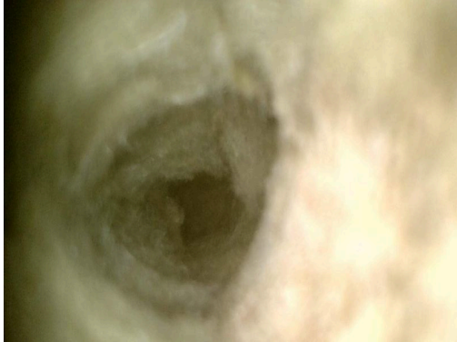
Photo indicators of filled cavity insulation:
