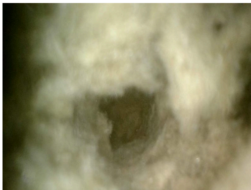
Photo indicators of filled cavity insulation:
