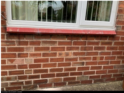
Photo indicators of filled cavity insulation:
