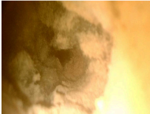
Photo indicators of filled cavity insulation:
