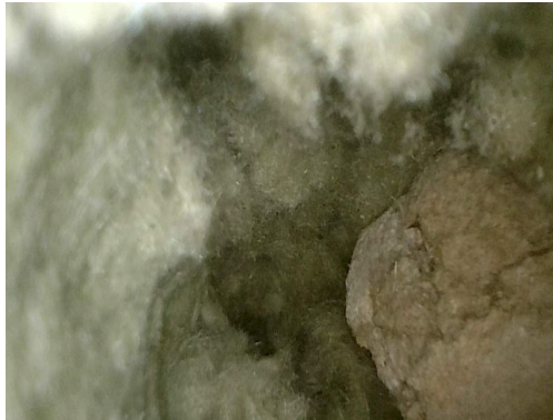
Photo indicators of filled cavity insulation:
