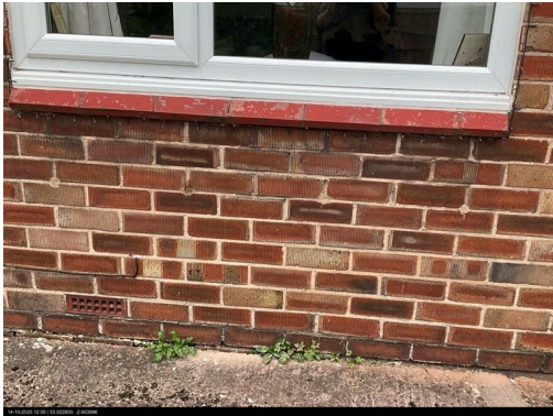
Photo indicators of filled cavity insulation:
