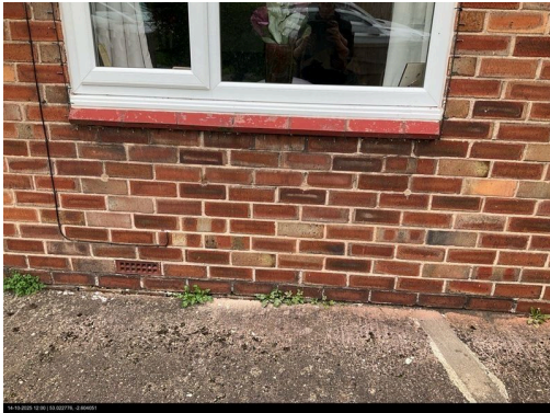
External indicators of Cavity Wall Construction:
