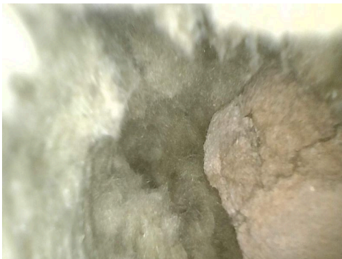
Photo indicators of filled cavity insulation:
