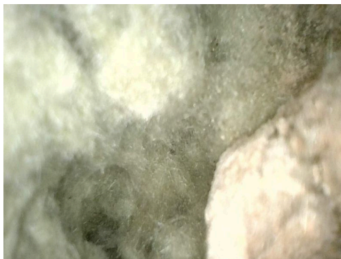
Photo indicators of filled cavity insulation:
