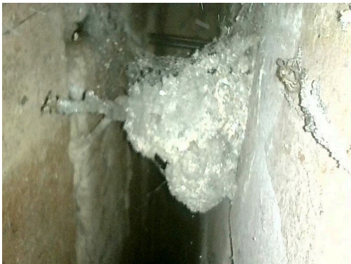
Photo indicators of filled cavity insulation:
