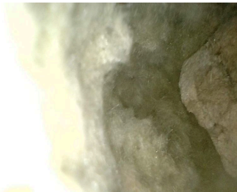
Photo indicators of filled cavity insulation:
