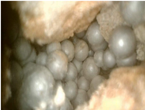
Photo indicators of filled cavity insulation:
