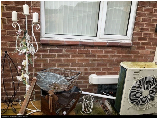
External indicators of Cavity Wall Construction:
