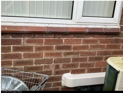
Photo indicators of filled cavity insulation:
