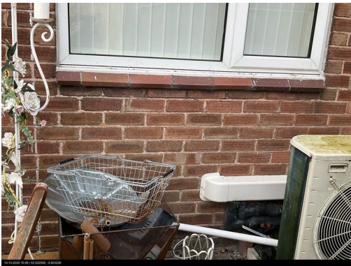
External indicators of Cavity Wall Construction:
