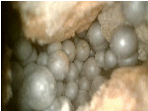
Photo indicators of filled cavity insulation:
