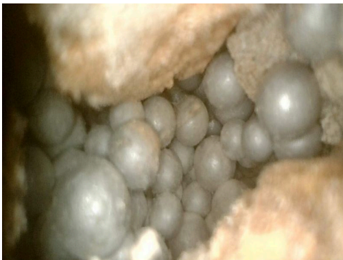
Photo indicators of filled cavity insulation:
