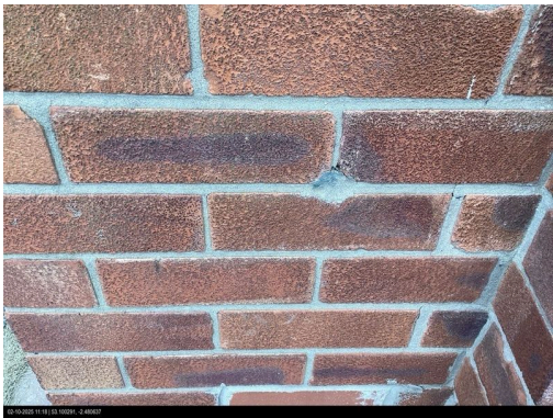
Photo indicators of filled cavity insulation:
