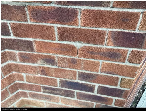
Photo indicators of filled cavity insulation:
