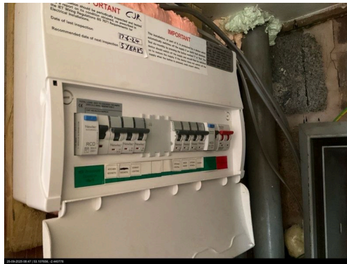
Photo of electricity meter:
